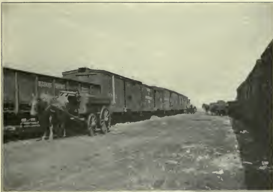
FIG. 52. MATERIALS IN TRANSIT, A SOURCE OF DUST. From cars set on team tracks, merchandise of many kinds is handled. The bare earth is stirred up by team traffic and the litter from materials handled accumulates.
